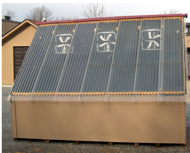
Figure 5. Front view of kiln showing fan placement.
